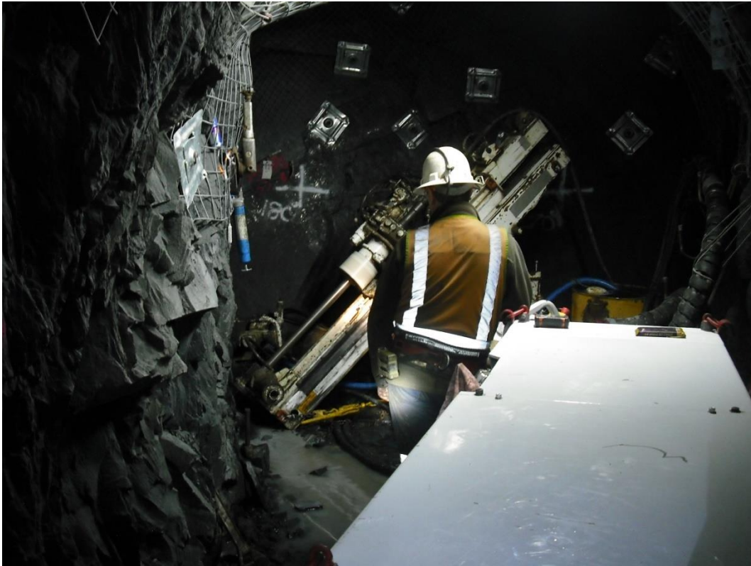
Figure 2: Diamond drilling – Rose of Denmark.
