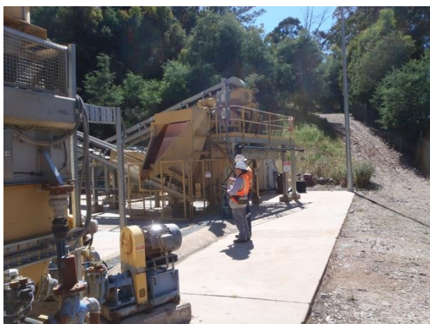
Photos 1 and 2: Inspection of plant for restart
