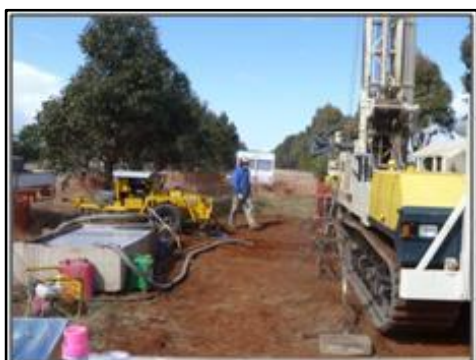
Figure 4: Drilling (hole MBM4).
